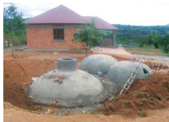
Photo: Wagga Wagga Primary School – Biogas during construction
