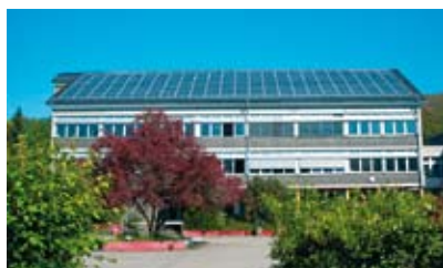
Photo: solar+spar contract GmbH – Aggertal High School
