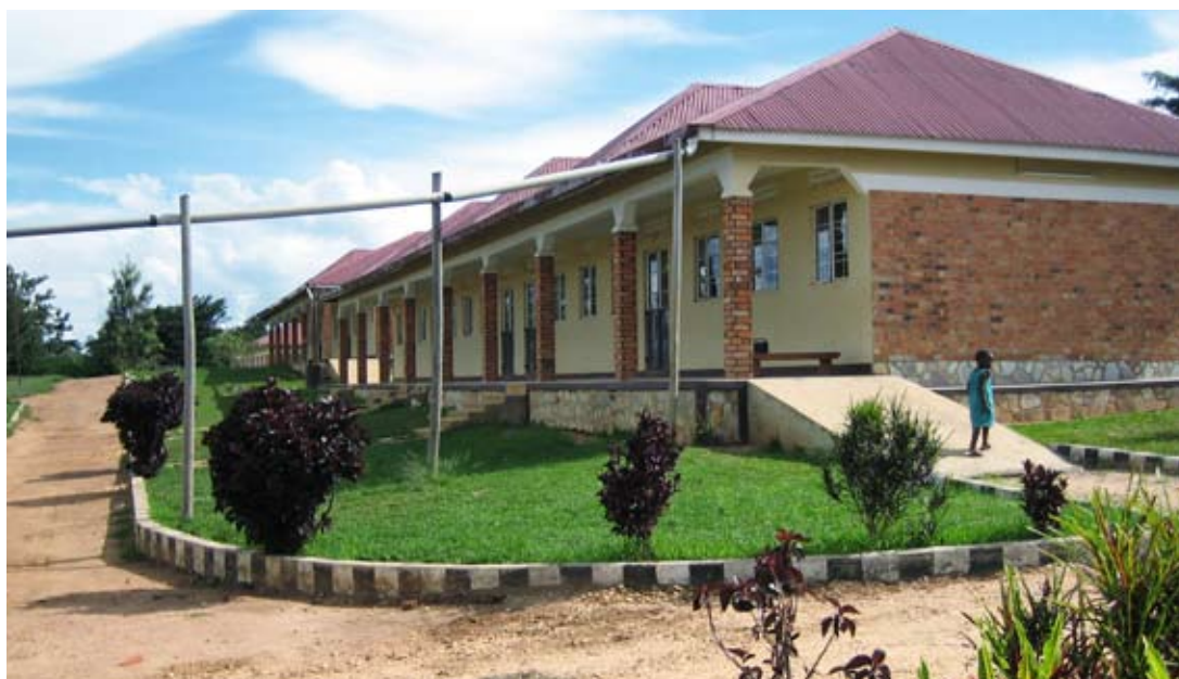
Photo: Wagga Wagga Primary School – Classroom blocks
