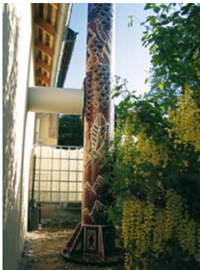
Photo: Ecole Ste Marie – The artistic face of the chimney
