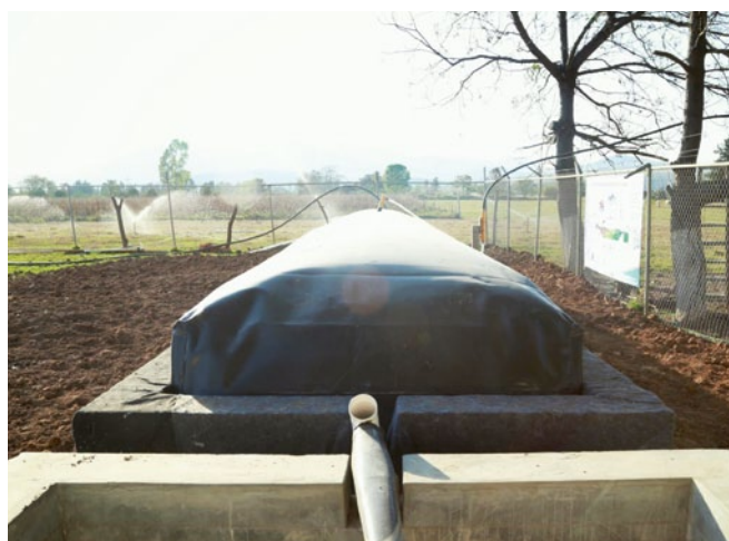
Examples of biodigesters installed by IIRI for the treatment of livestock waste in Mexico
