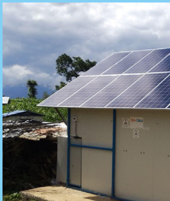
Cold storage unit in Baiteshwor after construction. (Photo: PEEDA, 2019)
