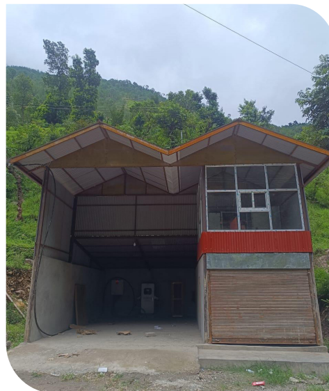
Figure 10: EV charging station under construction near Burtibang
